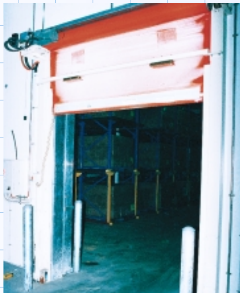
Special designs for freezers operating at - 30°C
